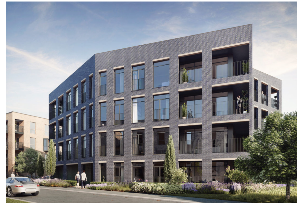
Barton Estate, Alison Brooks Architects
