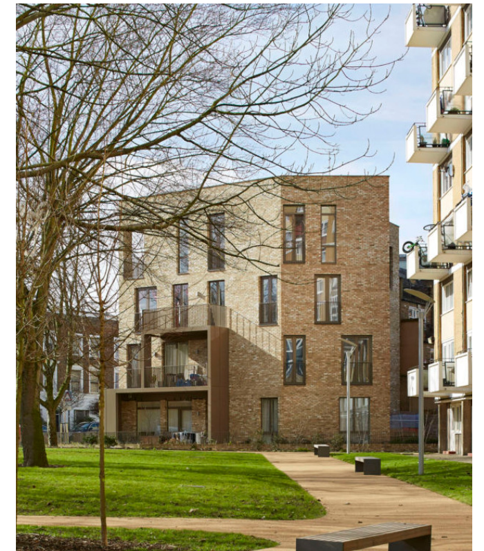
Ely Court, Alison Brooks Architects
